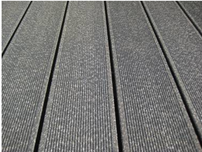
Close-up view of WPC decking
